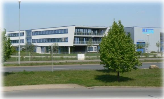
Minda KTSN Plastic Sol. GmbH & Co.KG Plant Location : Pirna, Germany Mexico (Upcoming)
